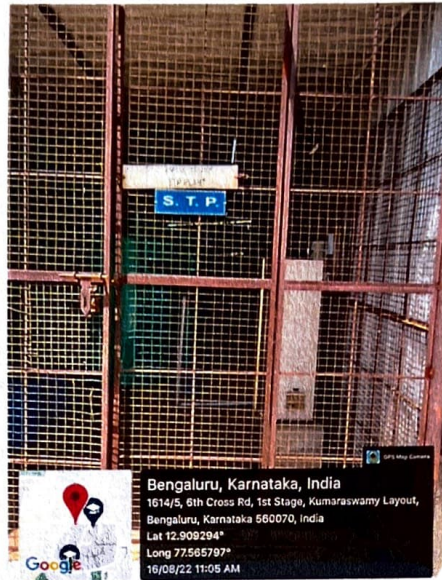
SEWAGE TREATMENT PLANT
